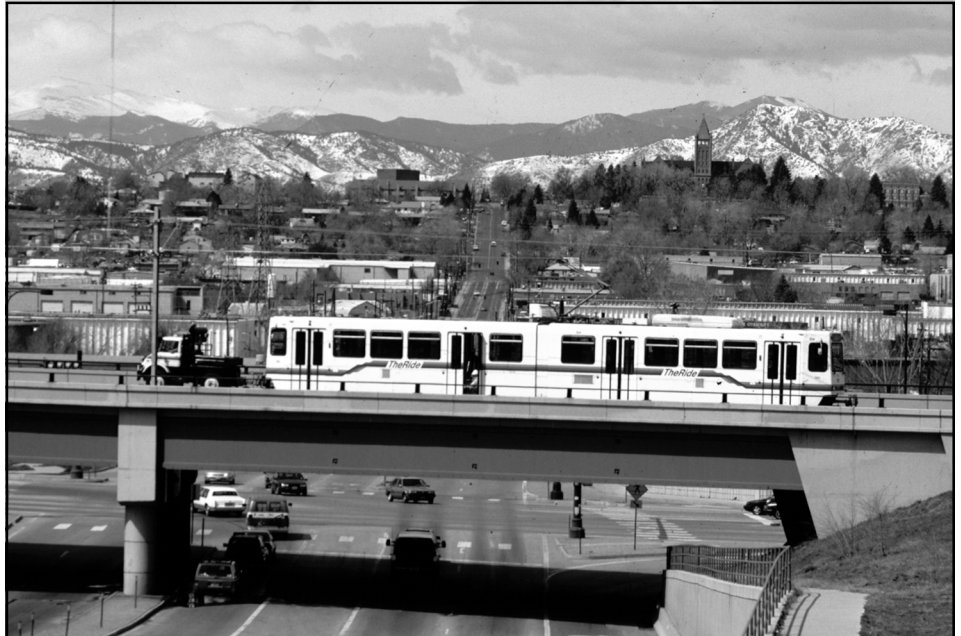
RTD's Light Rail Car No. 104 travels over Dartmouth Avenue on April 2nd. The car was towed south on the new route for clearance testing. The line is scheduled for its grand opening in July. – Photo © Darrell Arndt
